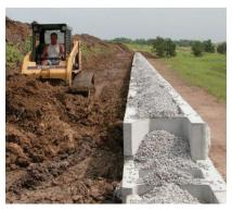
An internal drainage system is integrated into the wall through a void in the center of each Stone Strong block, no tubing to break or fail. The stone infill provides the drainage.
