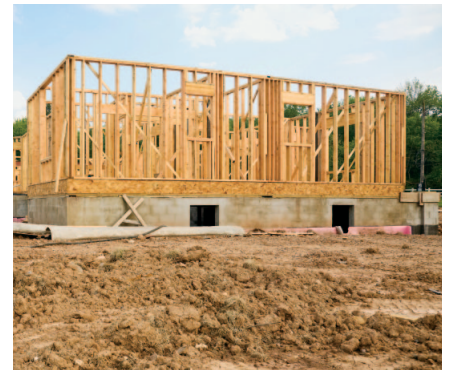
Our 3/4" round river rock meets residential radon mitigation requirements, Section AF103.2 of the Minnesota Residential Energy Code.
